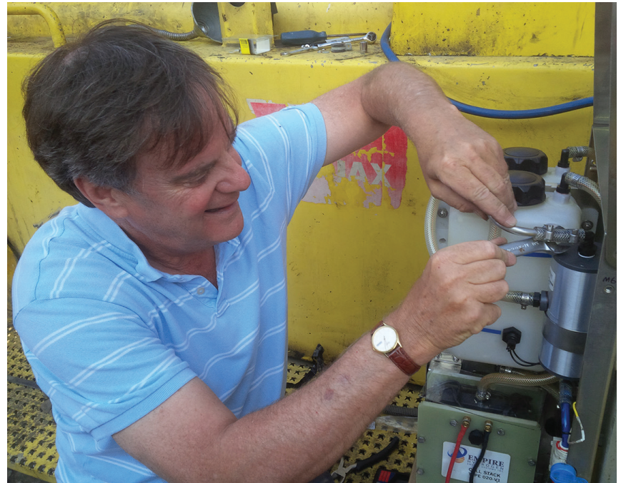
Executive Vice President Andrew Evans completes the installation on a container lifter in Surrey
